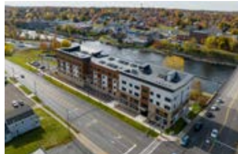
DePaul Lock 7 Apartments SWBR
