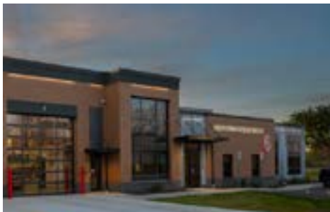
Henrietta Fire Department Fire Station No. 6 Passero Associates
